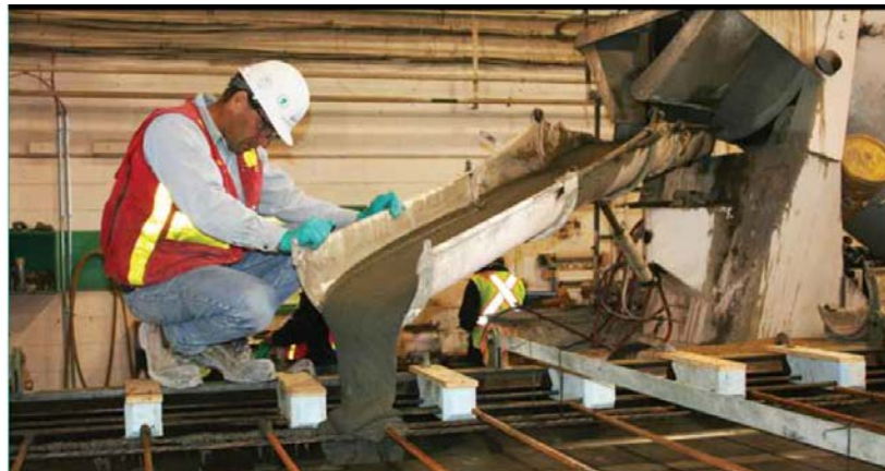
Figure 1.4 UHPC delivery (Graybeal, B., 2011)
